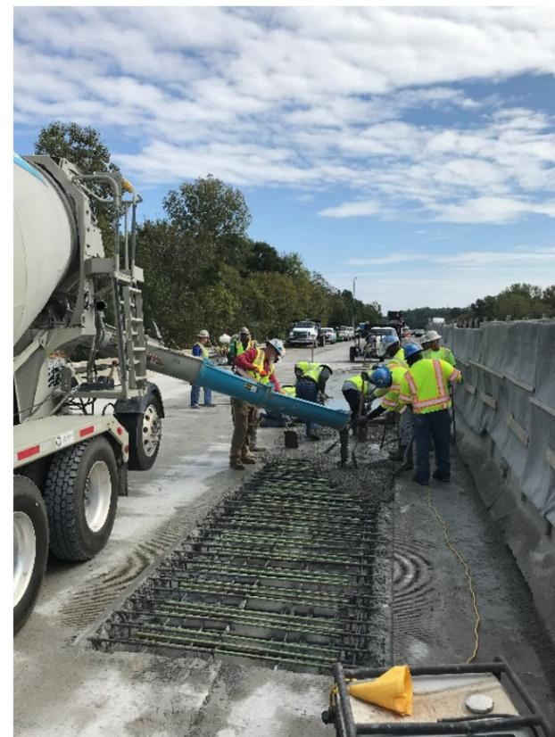
*Full depth deck repair (weekend lane closure - hydro concrete demo)*
