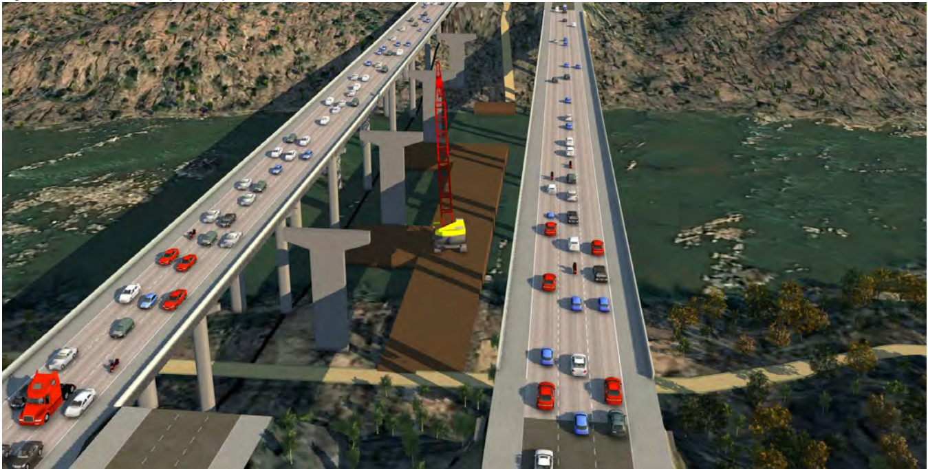
Figure 4.7.1.4 - Causeway with Open Channels at All Times
