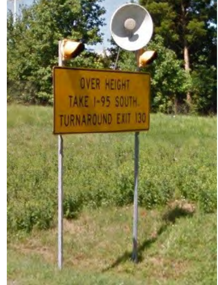
Figure 4.5.2.3 - Existing Overheight Detection System will be relocated and maintained.
