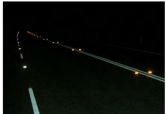
Figure 4.5.2.9 - Raised Pavement Markers
