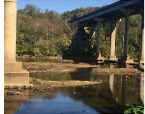
Figure 4.4.3.2 - Rappahannock River Bed Existing Condition during low-flow
