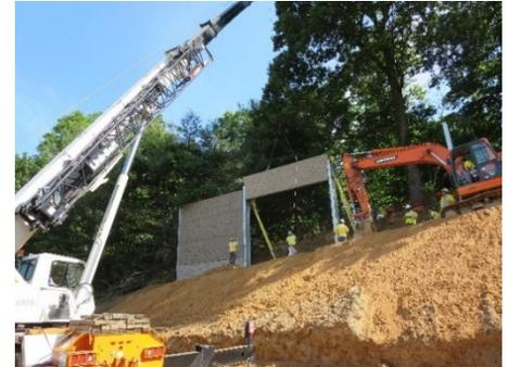
*Figure 4.5.1-6. LANE’s I-66 WB (Spot Improvements project) also included noise barrier installation.*
