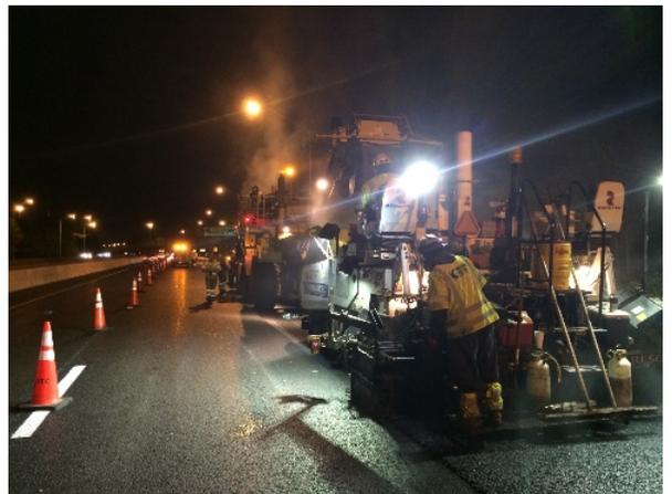
*Figure 4.5.1-7. Milling and paving will be performed overnight to minimize impacts to the traveling public.*
