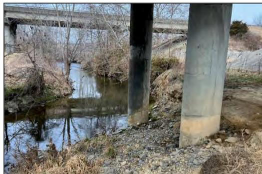
*Figure 4.3.2-5: Lewis Creek Existing Scoured Condition*
