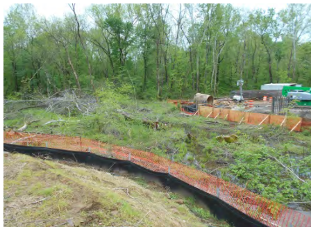
Figure 4.4.1-5 – Install Exclusion Fencing to Protect Non-Impacted Wetland Area
