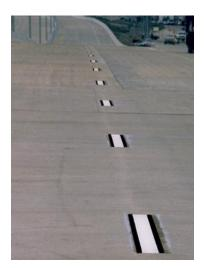
new (whiter) concrete than aged concrete, both for "normal" drivers and for vehicles that attempt to sense the edge lines and lane lines for lane departure avoidance systems.
