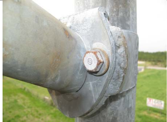
Weld around upper chord to mounting plate connection 50% complete
