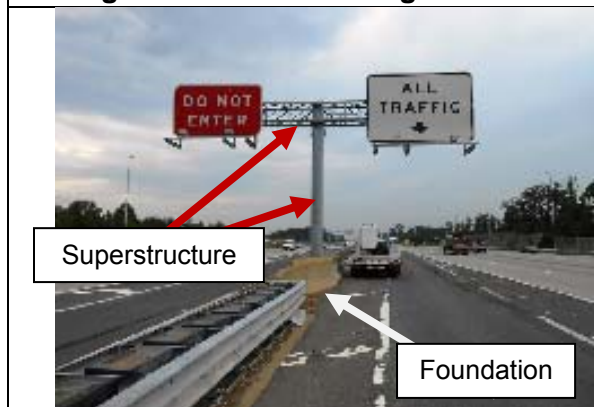
Figure 1 – Cantilever Sign Structure
