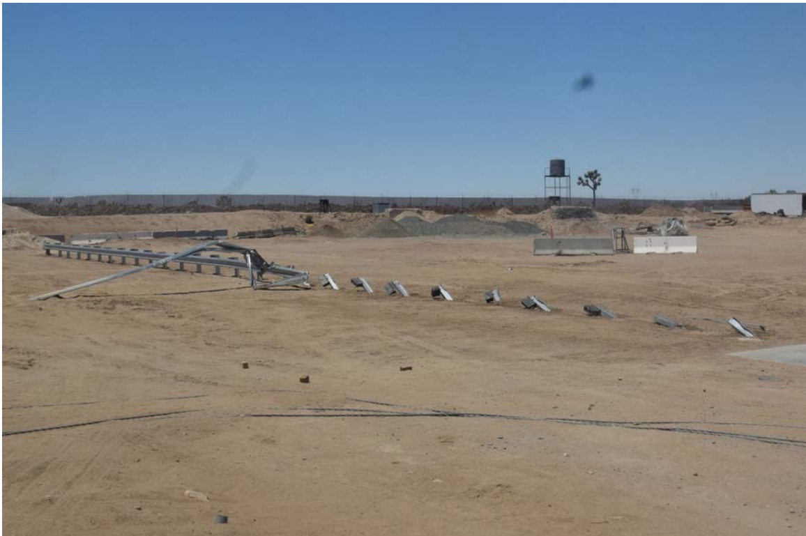
FIGURE 20. Post-Test Right Front \frac{3}{4} View of Test Article
