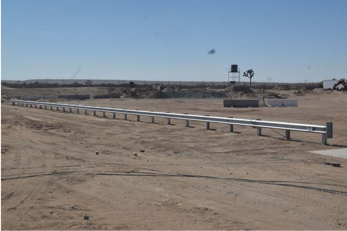
FIGURE 19. Pre-Test Right Front \frac{3}{4} View of Test Article
