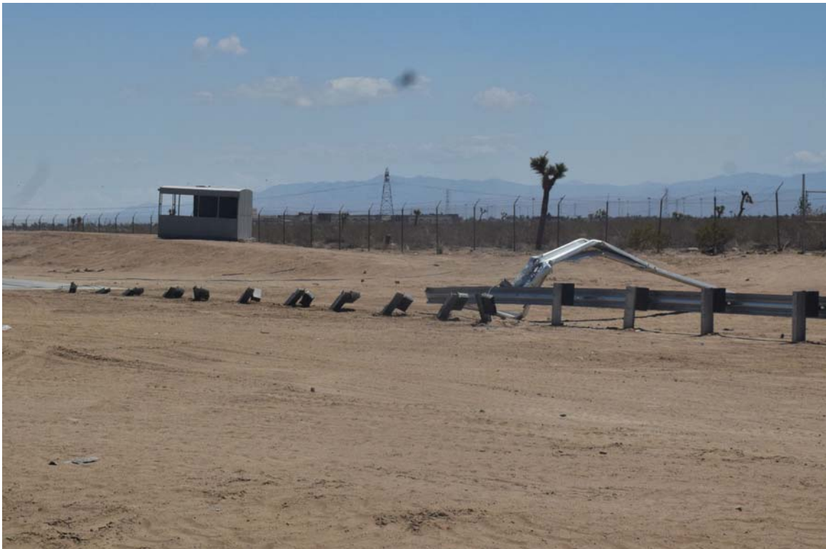
FIGURE 28. Post-Test Left Rear \frac{3}{4} View of Test Article
