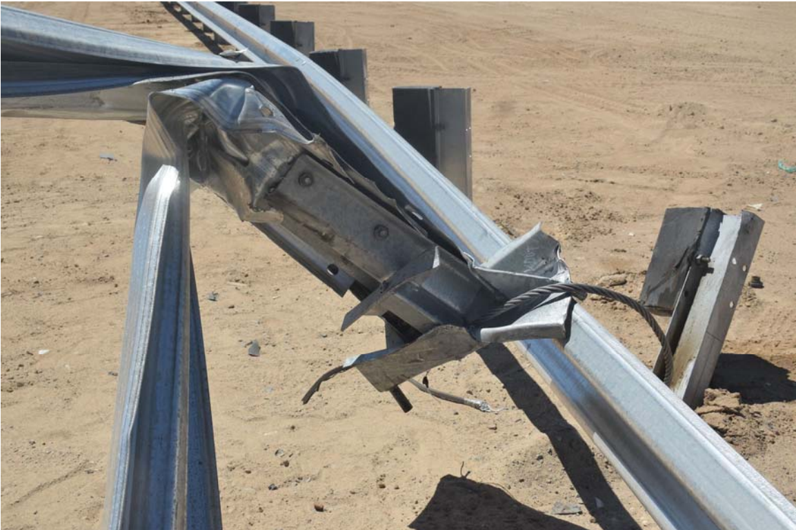
FIGURE 38. Test Article Damage
