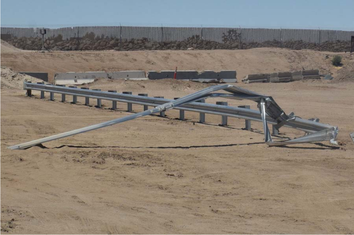
FIGURE 37. Test Article Damage
