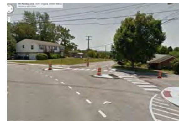
Figure 2: Traffic calming islands were completed first at Harding Elementary School in Blacksburg
